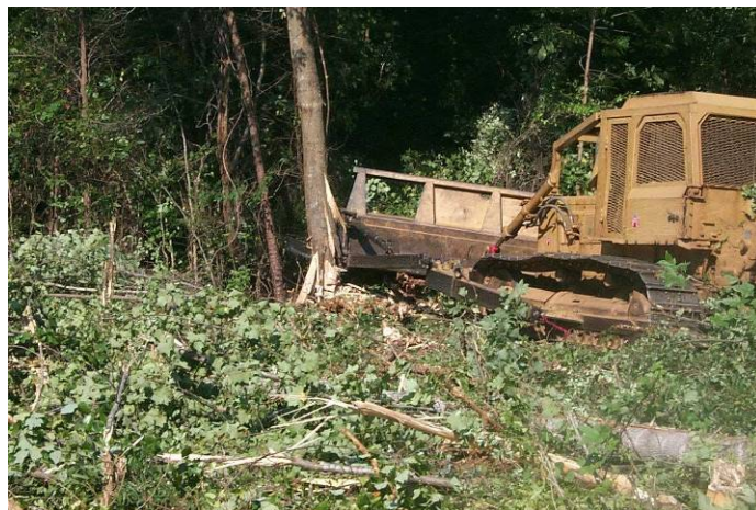
KG-blade used for shearing during site-prep.
